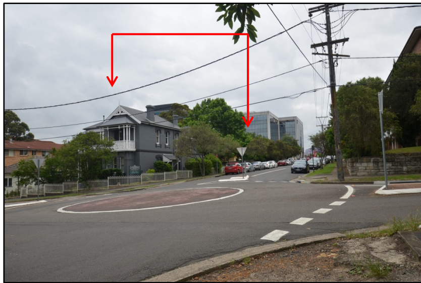
Figure 16. View towards the subject site from the intersection of Harold and Sorrell Streets. The extent of the site is indicated by the arrows. (Source: Heritage21, 11.11.15).
