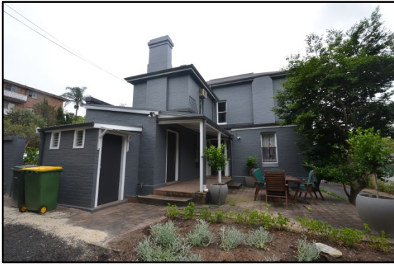
Figure 35. Western façade of the Currawong house. (Source: Heritage21, 11.11.15).
