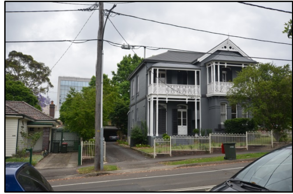
Figure 18. Sorrell Street frontage of the heritage item I420. Note multi-storey development in background. (Source: Heritage21, 11.11.15).
