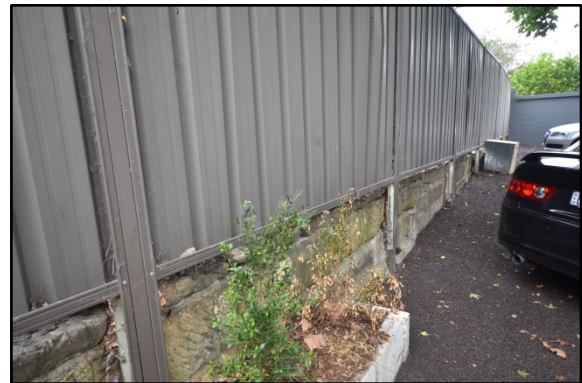
Figure 44. Sandstone wall located along the northern boundary of rear section of Currawong house. (Source: Heritage21, 11.11.15).
