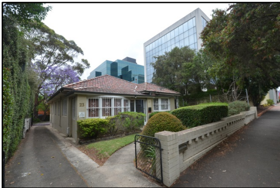
Figure 21. View of dwelling located at 23 Harold Street, adjacent to multi-storey development. (Source: Heritage21, 11.11.15).
